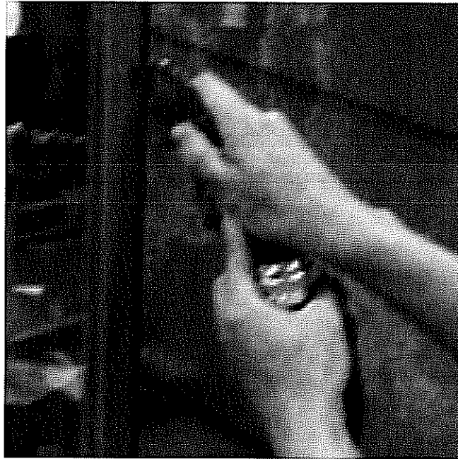
Figure 6 – Wedge Cutting IG Sealant
