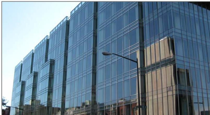
Tony D'Agostino, Principal and Project Manager of RTKL Associates, Inc., responded, "The performance criteria for the glass was of utmost importance given the all-glass design of the building. We conducted research on a wide variety of glass types which would give us the performance we needed and, at the same time, give us a clear non-reflective aesthetic without tints and without the upcharge for low iron. Solarban 70XL best achieved both." Providing a solar heat gain coefficient (SHGC) of
